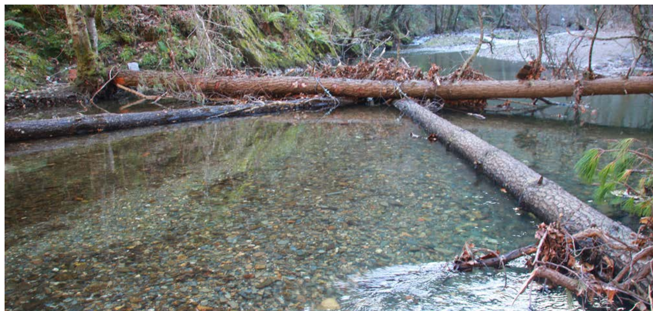
Riverbed restoration with wooden structures | Hazi
